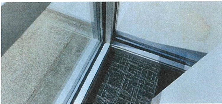
Photo 3-1 West entry / exit.
